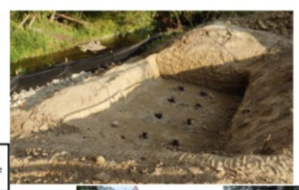
The framing on top of the Helical Piles now ready for the first concrete to
