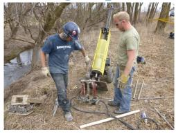
Core samples from 30 feet down were taken and determined that the ground is mostly clay. The result is a new modified abutment design to stabilize the bridge in unstable soil. The soil findings have delayed the project slightly, but the township is moving ahead with sourcing a bridge builder.
